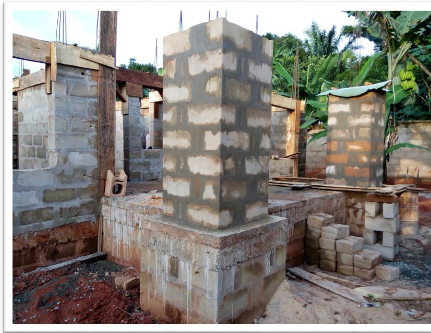
Figure 79: Blockwork in progress at Project 'B' site as at December, 2019.
