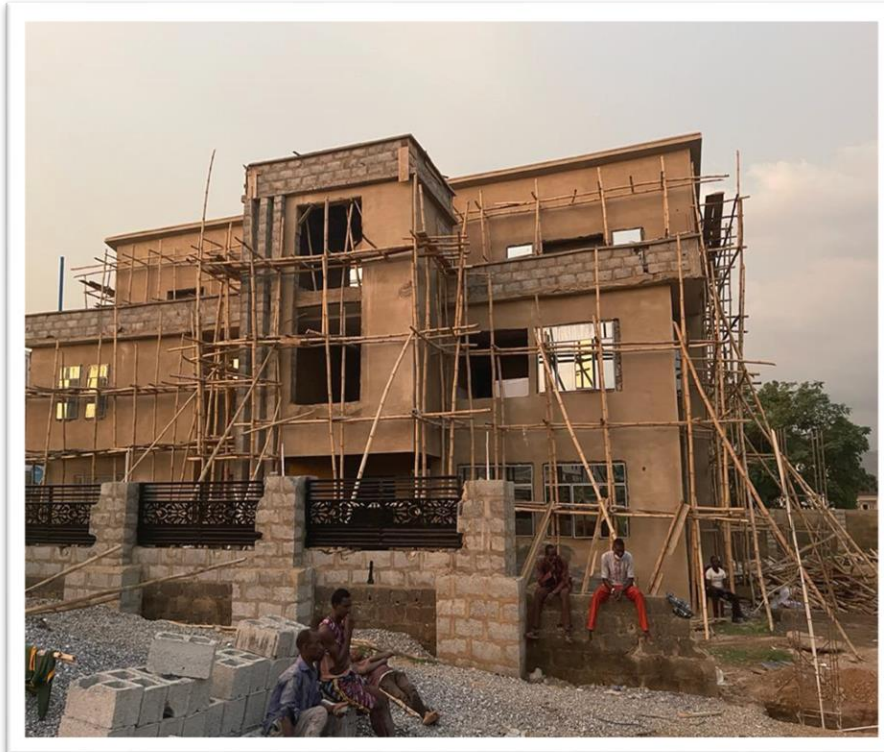
Figure 47: Plastering and fixing of windows in progress. The same goes for some level of brickfacing on the parapet wall.
