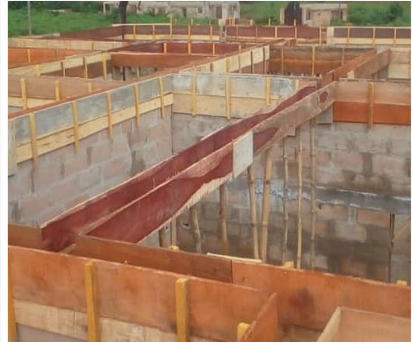
Figure 78: Almost at the +4.050m levels with the formwork of the r.c. beams in place as at January, 2020.
