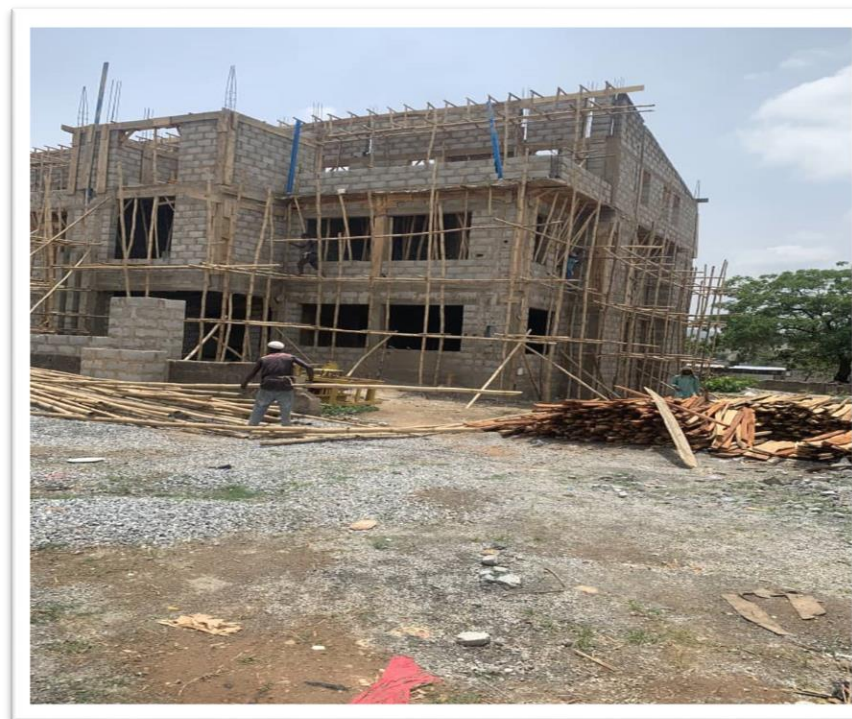
Figure 50: Blockwork in advanced stage.
