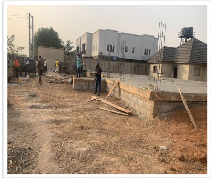
Figure 45: Casting of oversite concrete has reached near completion. The project architect can be seen issuing instructions to the labourers. This candidate is the photographer.
