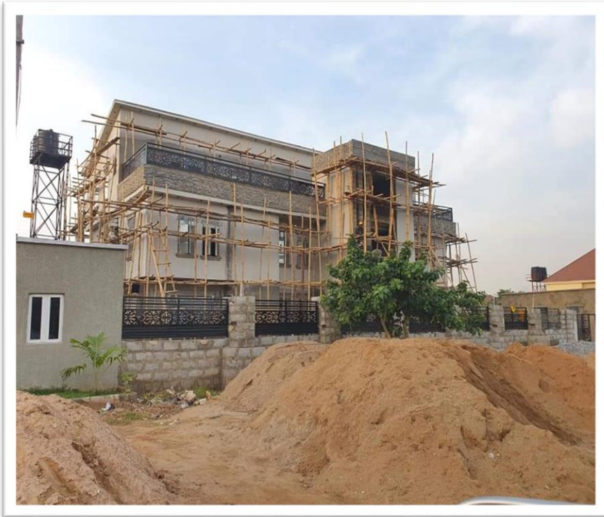
Figure 49: Handrails have been fixed, plastering near completion and window architrave fixed.
