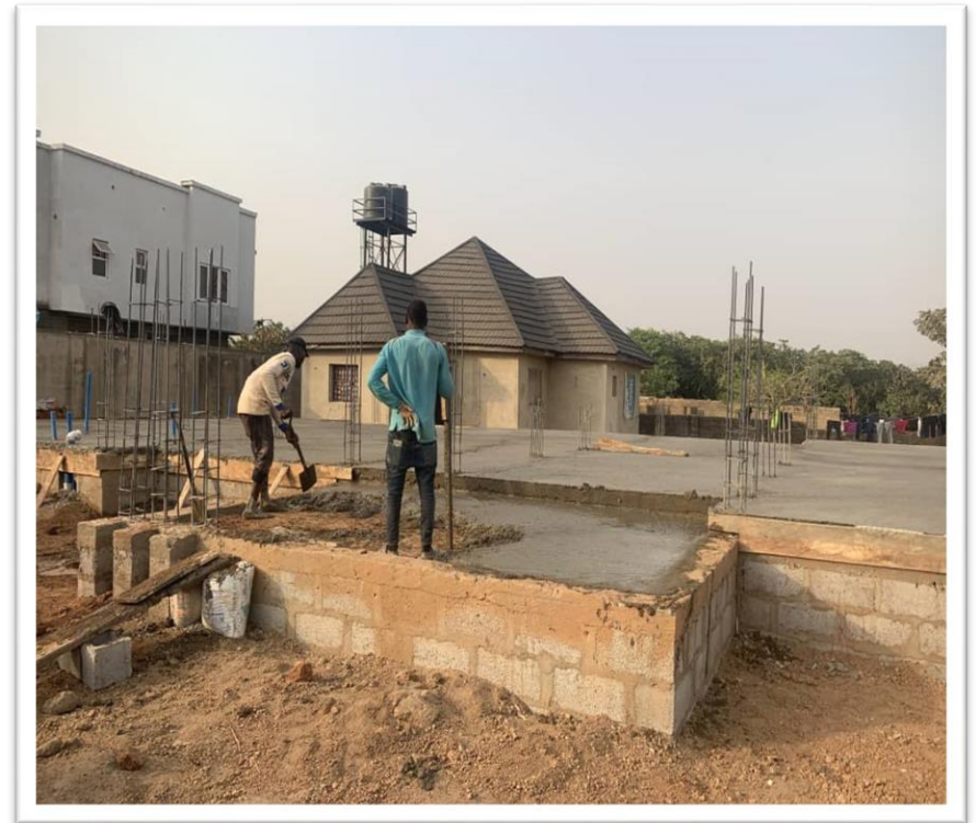
Figure 46: Placement of the 150mm thick oversite concrete.
