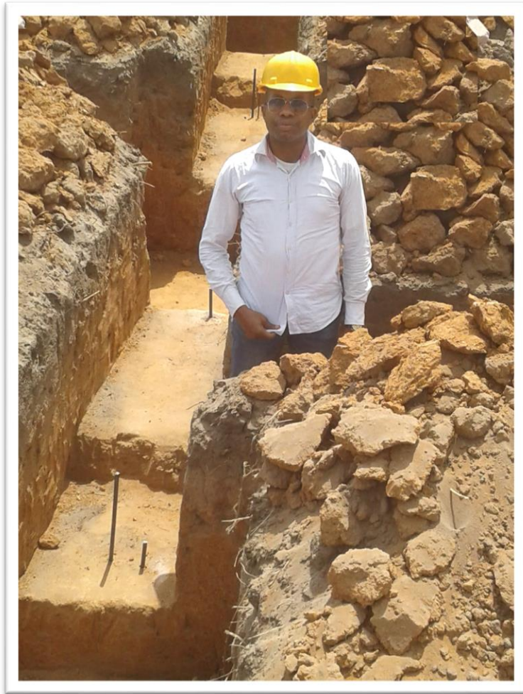
Figure 77: Excavation stage: The foundation was stepped to compensate for the sloped site.
