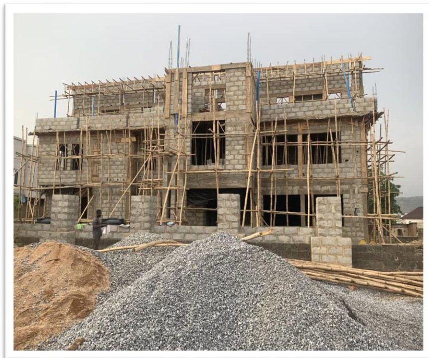
Figure 51: Blockwork and fencing in advanced stage.
