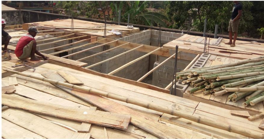
Figure 81: Boarding in preparation of the r.c. first floor deck. As at January 2020. At this time, the COVID-19 pandemic has started affecting vehicular movement.
