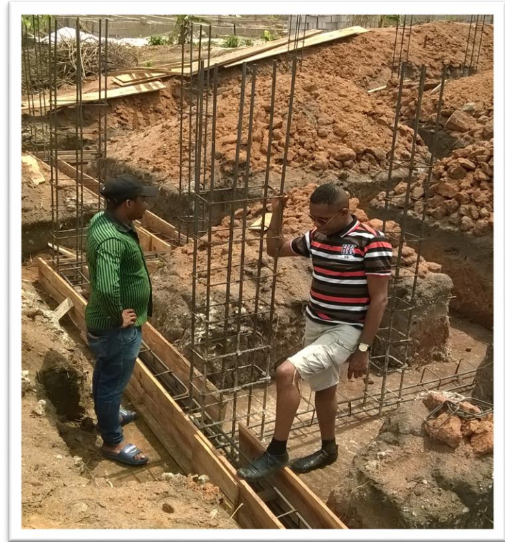
Figure 76: Adhering to the consultant structural engineer's instructions: Boarding for the r.c. 225mm X 225mm underground beams. The resident architect checks for proper alignment of rebars.
