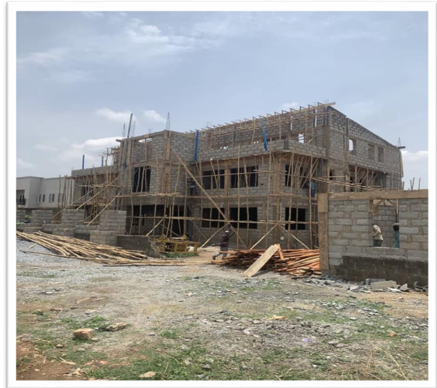
Figure 48: Another shot of the blockwork in advanced stage.
